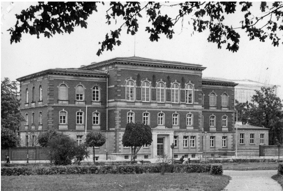
The new home in Würzburg: The former officers' mess of the 9th Bavarian Infantry Regiment is being converted for the Max Planck Institute – on the right, the first glass melting hall © Max Planck Society
